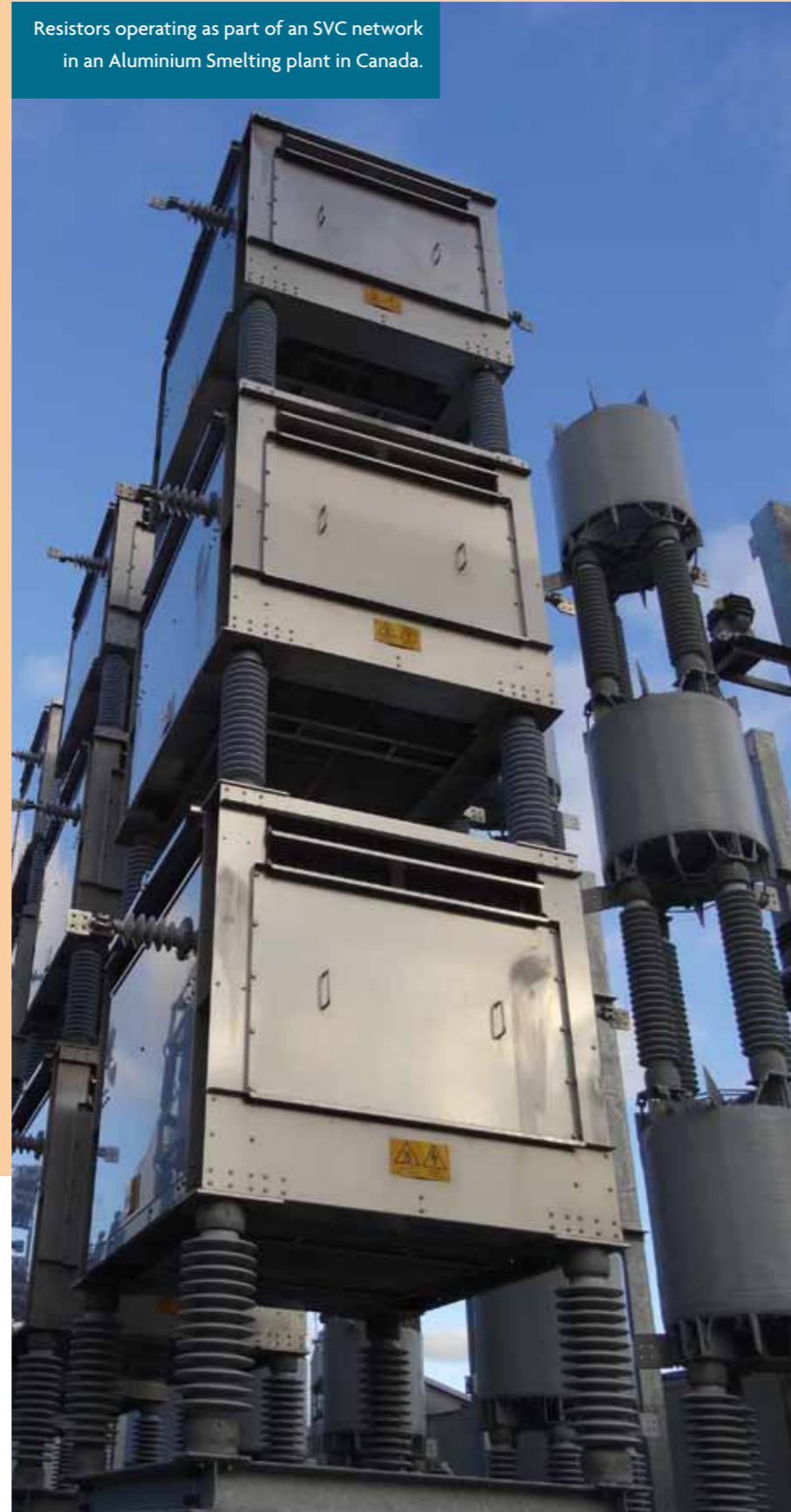
High voltage filter resistors with snow stands installed in Canada
